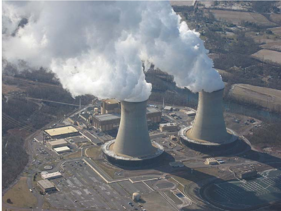
Limerick Generating Station in Limerick, Pennsylvania
