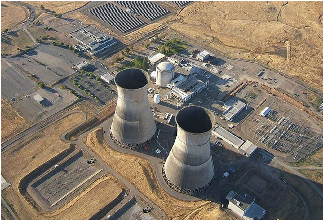
Rancho Seco Power Plant in Herald, California
