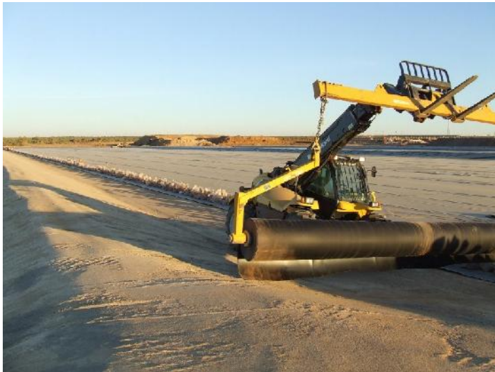
Pond liner installation, photo courtesy GDT Lining
