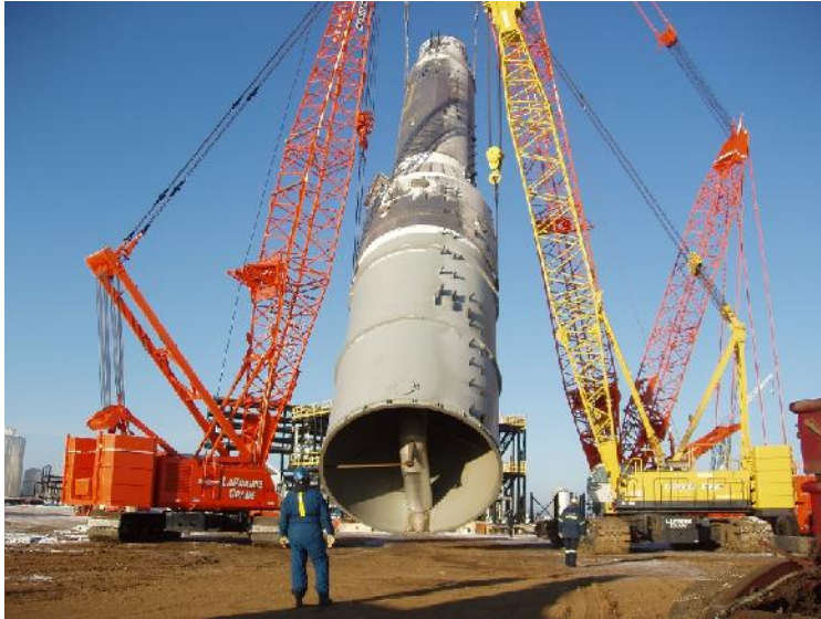
Evaporator installation, photo courtesy MarketWatch.com
