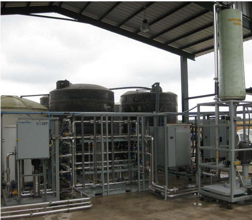
The VSEP system is currently treating approximately 140 m<sup>3</sup>/day of leachate from their storage ponds. VSEP systems are modular, so expansion is easy at any time. This will allow for plenty of storage capacity and will allow for time to select the best disposal method for the concentrated leachate that remains.
