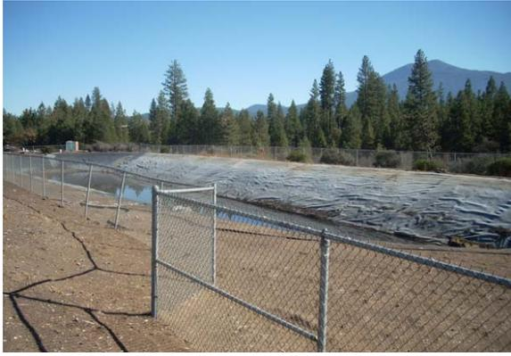
corrosion-resistant materials. Evaporation ponds must be lined and may not be feasible in locations with limited space and low net evaporation rates; furthermore, no water is reclaimed in the process.
